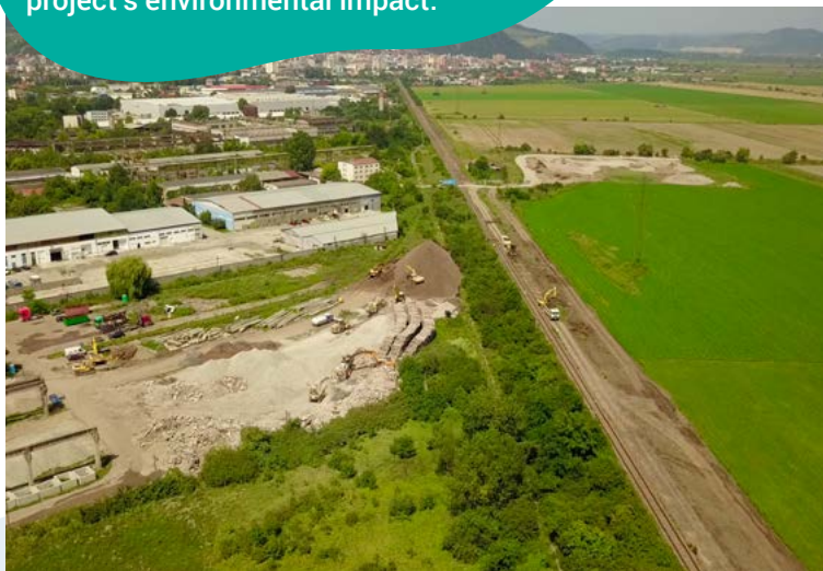
Platform for crushing cement from the demolition of the superstructure
